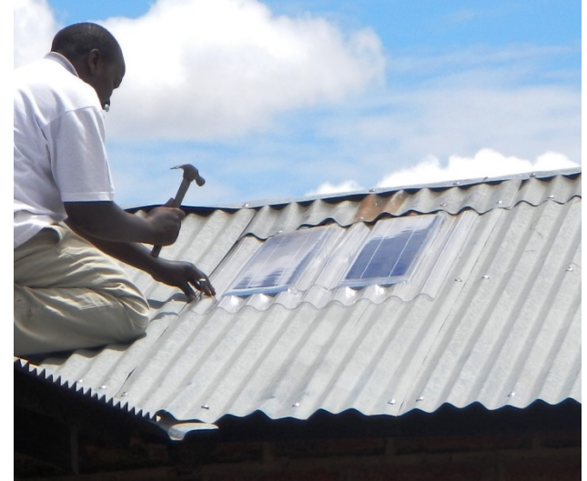
Solamander 36 W photovoltaic panel mounted on a corrugated roof and held in place with nails
