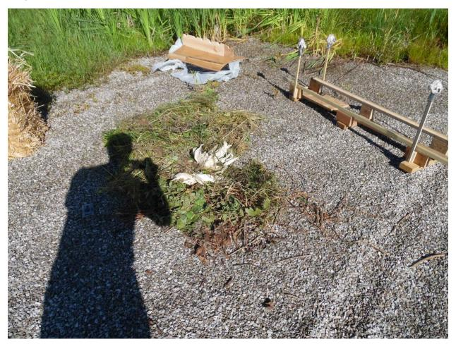
About 5 cm of loose insulation. Here, I started with weeds and corn husks, then added straw to build it up to 5 cm thickness.
