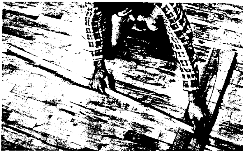
Photo 5-1—Draw the 53-inch gusset radius, using a shop-made compass pivoting from the floor.
