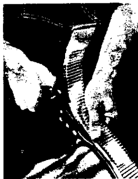
Photo 7-2—Carefully cut the stovepipe to length with a tin shears. Be very careful of the sharp edges.
