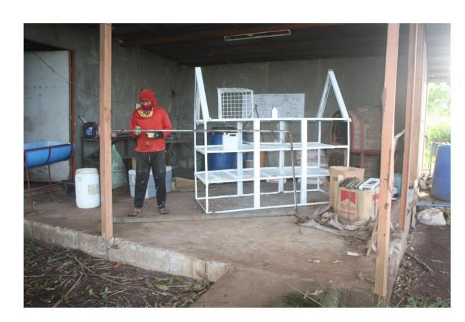
A concrete foundation was constructed on which the dryer was laid over. This concrete floor was embedded with the plastic garbage and broken glasses of the farm which has already become irritating and poses hazards to the workers.
