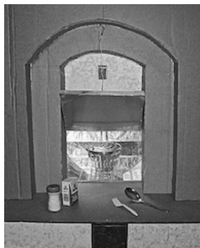
Through-the-wall kitchen solar box cooker. Courtesy of Joel Goodman 2013
