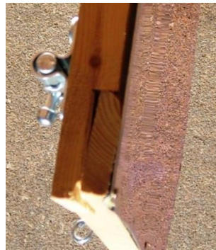
Detail at reflector wood oven door and ferrocement frame
