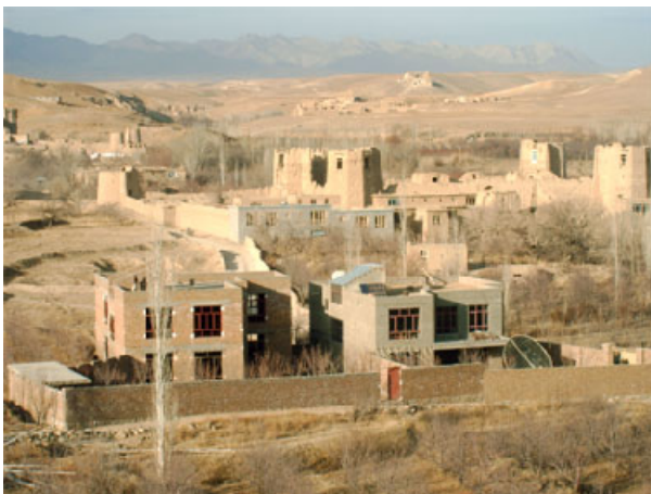
Picture 2 : new primary school (left) and Center for Renewable Energy (right)
